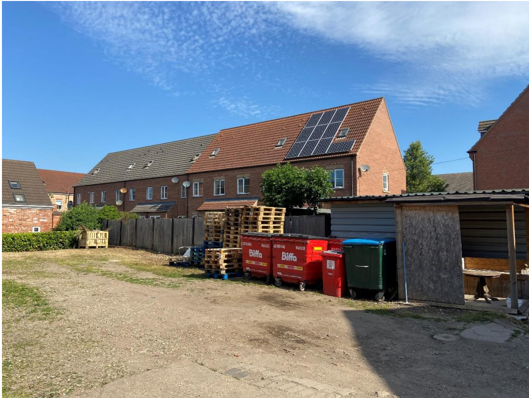
Anchor Close properties to the north
